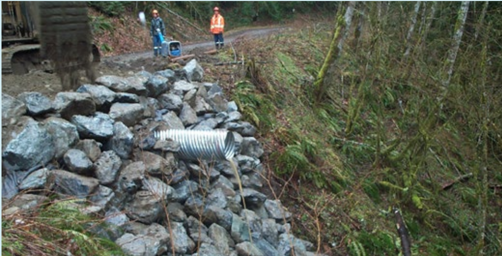
Repairing a culvert embankment armoured with rock. Photo credit: FLNRO
