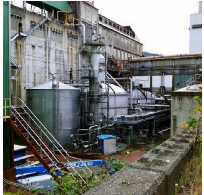
Neucel pulp mill facility in Port Alice Source: Environmental Emergency Program
