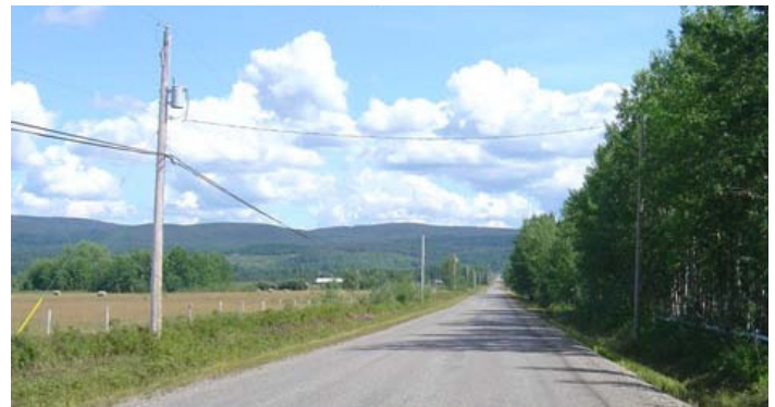
Sealcoating (applying a layer of bituminous material to a road surface to seal it) is a commonly used maintenance technique applied to many secondary roads in British Columbia. - Auditor General staff photo
