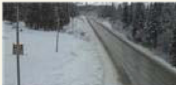
Web cam image of Pine Pass on Highway 97, north of Mackenzie Junction at Powder King access road, looking north (Source: www.drivebc.ca/ )
