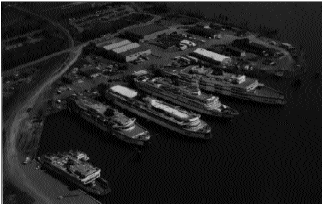
Deas Dock Refit Complex
