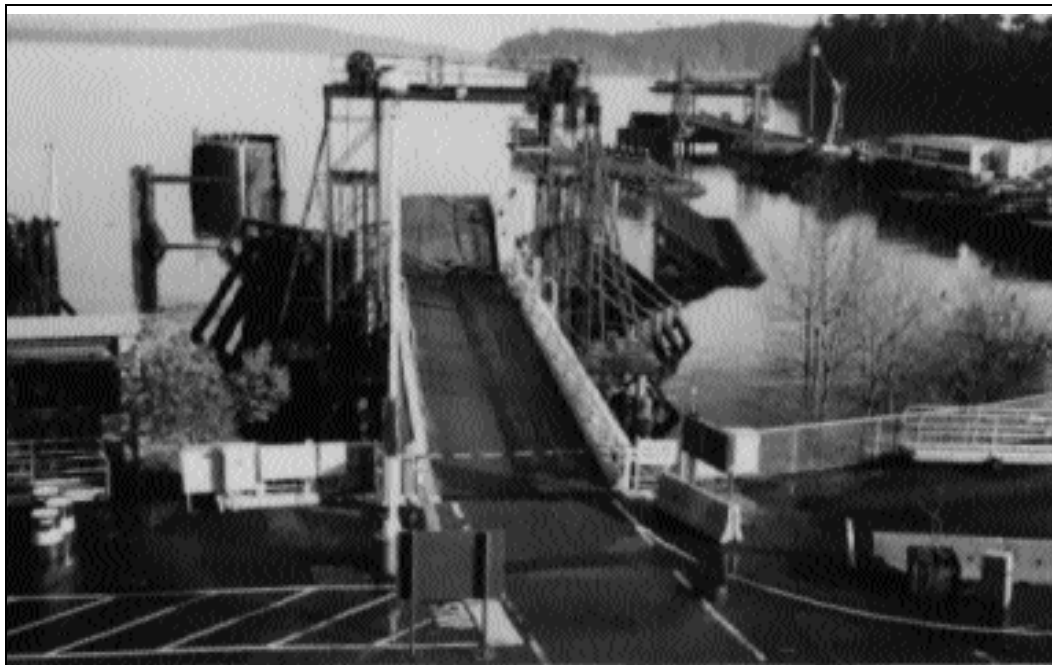
Single lane ramp built in the late 1960's at Swartz Bay
